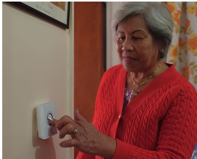
(Barnet Homes resident using Ei450 test switch)
