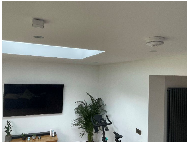
(The Environmental Sensor and Multi-Sensor alarm in situ)
